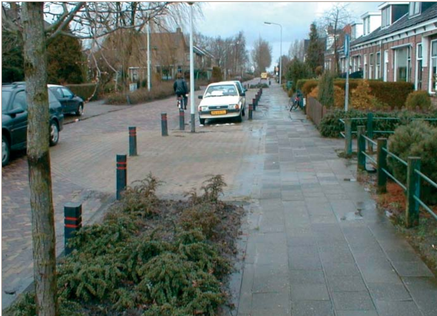
Fig. 12. Open footpath-road junction at Makkinga, Netherlands—motorists have their attention drawn to it by a change in surface treatment and a slight rise in road level
