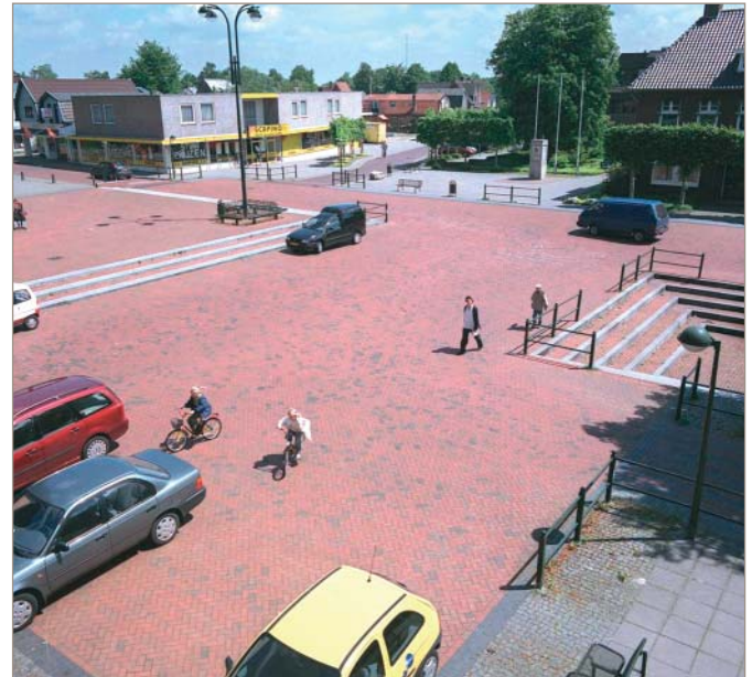
Fig. 11. The complex de Brink road junction in Oosterwolde, Netherlands has been converted to a shared public square without road markings or signs
